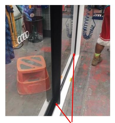
7. Adjust the rollers at the bottom of the panel so it lines up with the jamb when closed. Clockwise to raise. Anti-clockwise to lower.
