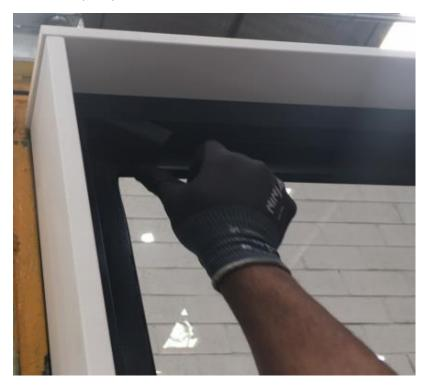
6. Fitting the sliding panel from the inside, rest it on the ground in front of the opening. Lift up and into the Head track then guide the bottom back in towards the sill until it is inside the frame then lower it onto the track. 2 people may be required.
