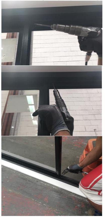
4. Using the Black 6g x 13mm screws, screw fix through the jamb and into the fixed panel (top, centre and bottom). Careful not to let the driver slip as damage may occur to the paint or frame.
