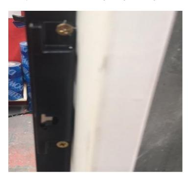
11. Fit the cover and install 2 x screws.
