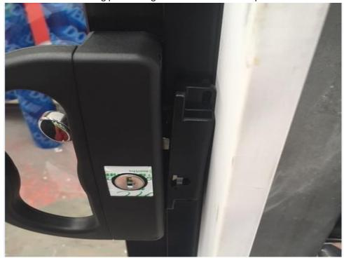
9. When the lock has been fitted, close the door, hold the keeper against the lock body and engage the parrot beak to hold the keeper in place.
