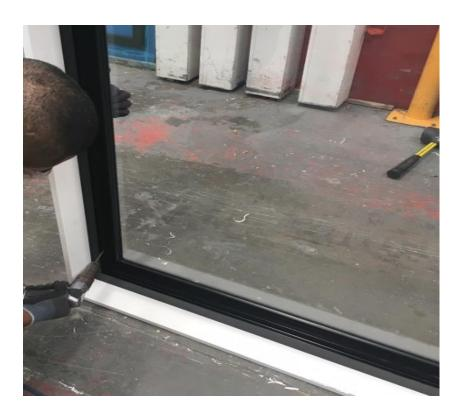
5. Make sure the Bump stop is still fitted in the head and has not fallen out during transport.
