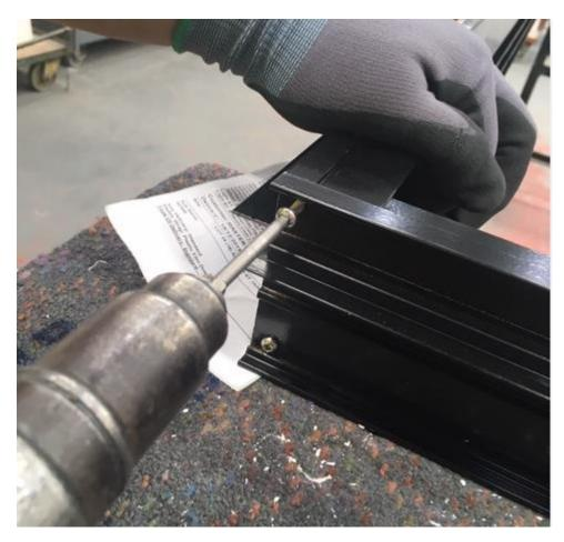
2. When the frame has been screwed together you can install it into the opening making sure it is square. Insert the fixed panel (from the outside) by lifting it into the head and pushing it in at the bottom where it will rest in the centre of the sill.
